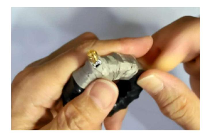
Wrap another layer of PCV insulation tape tightly to the ferrite core to secure the shielding in place properly
